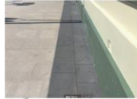
Bluestone paving strip to building facade
