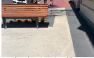
Shot blast finish concrete as main pavement body
