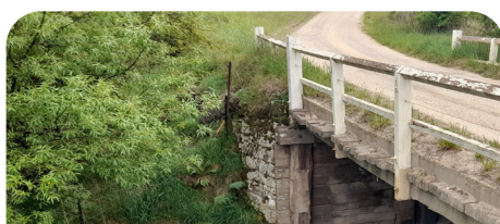
Bridge Replacement Program $1,066,303
